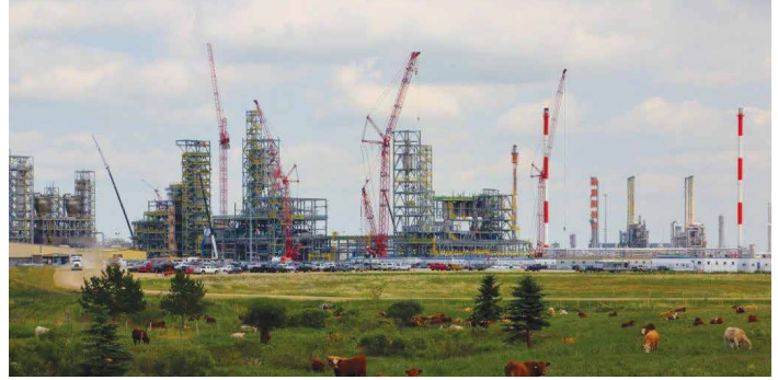
Main structures are substantially complete on our PE1 Expansion Project. Building cladding will soon be underway in preparation for Winter work.
